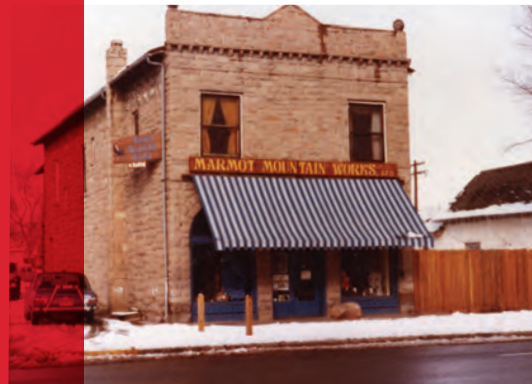
The first Marmot store in Grand Junction, CO
